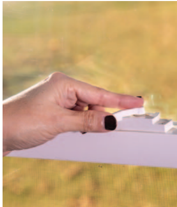
When checking your windows, ensure sash locks are installed properly and sealed tight when locked. Photograph by Mark Gilliland, Pioneer Utility Resources
