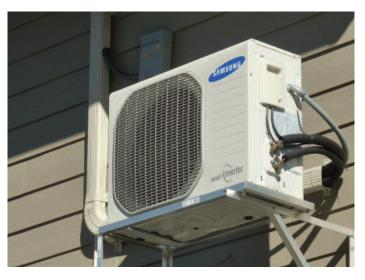
The condenser unit for a mini-split heat pump system is usually mounted on an exterior wall. Photograph by Gary Cziko
