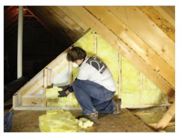
Some do-it-yourselfers are comfortable tackling an attic insulation project. The steep pitch of this roof and the plywood decking this person is kneeling on makes this project appear easy, but in most homes, you'll only be able to stand on the floor joists or rafters. Photograph provided by The EnergySmart Academy
