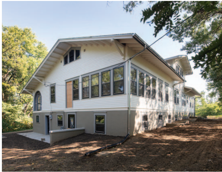
The building renovation project includes space for youth activities, a Native arts gallery and a gift shop. Photograph by Kurt Johnson
