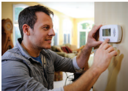
A programmable thermostat can help you reduce energy use when you don't need to be heating or cooling your home. Photograph by Consumers Energy
