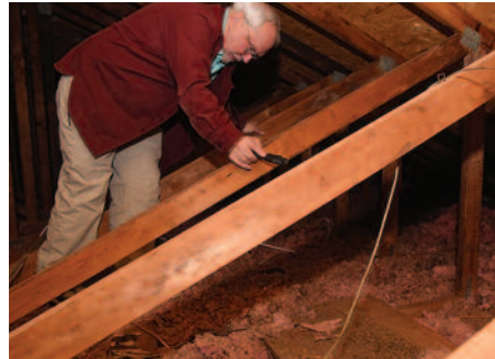
An auditor inspects insulation in the attic of a single family home. Photograph by Andy Harper, 60iMedia Productions
